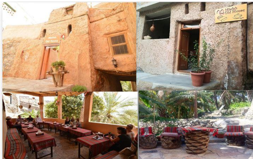
Figure 3: Misfat Old Village
